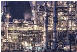
An example petrochemical processing plant. Grangemouth, Scotland. CC Public Domain. Source: pxhere.com.
